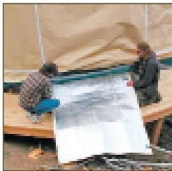
Wall insulation comes in panels that overlap approximately six inches. The panels are installed between the lattice wall and the exterior wall fabric.
