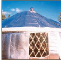
The roof insulation includes a separate lining that is visible above the rafters and conceals the actual insulation. The insulation itself goes between the lining and the exterior roof.
